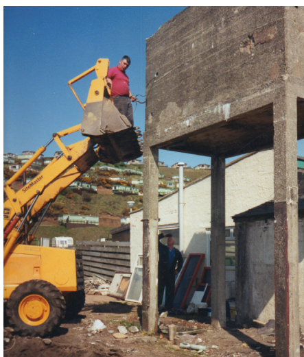
Commencing the demolition of the old water tank.
